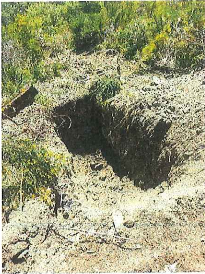
Photo 4 – Test pit near the Toe
