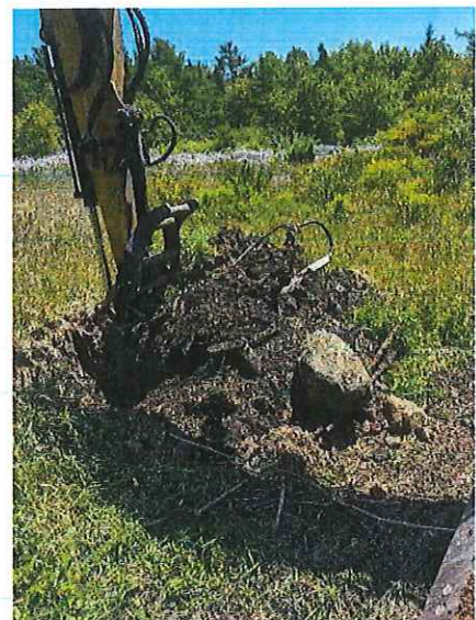
Photo 3 – Test Pit on Top
