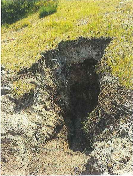
Photo 2 – Test Pit on Side Slope
